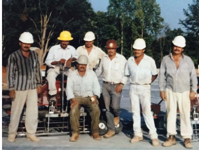
Figure 10. Hermanos Valdez, Christian's father, grandfather, and five uncles on a paving job site. Pictured (from left to right) are Leopoldo Valdez, Jesús Valdez (grandfather, yellow hardhat), Jesús Valdez, Jr. (next to grandfather on the right), Martín Valdez (gray hardhat), Ernesto Valdez (father, brown hardhat), Orasmo Valdez, and Felix Valdez (white hardhats). All permissions granted.
